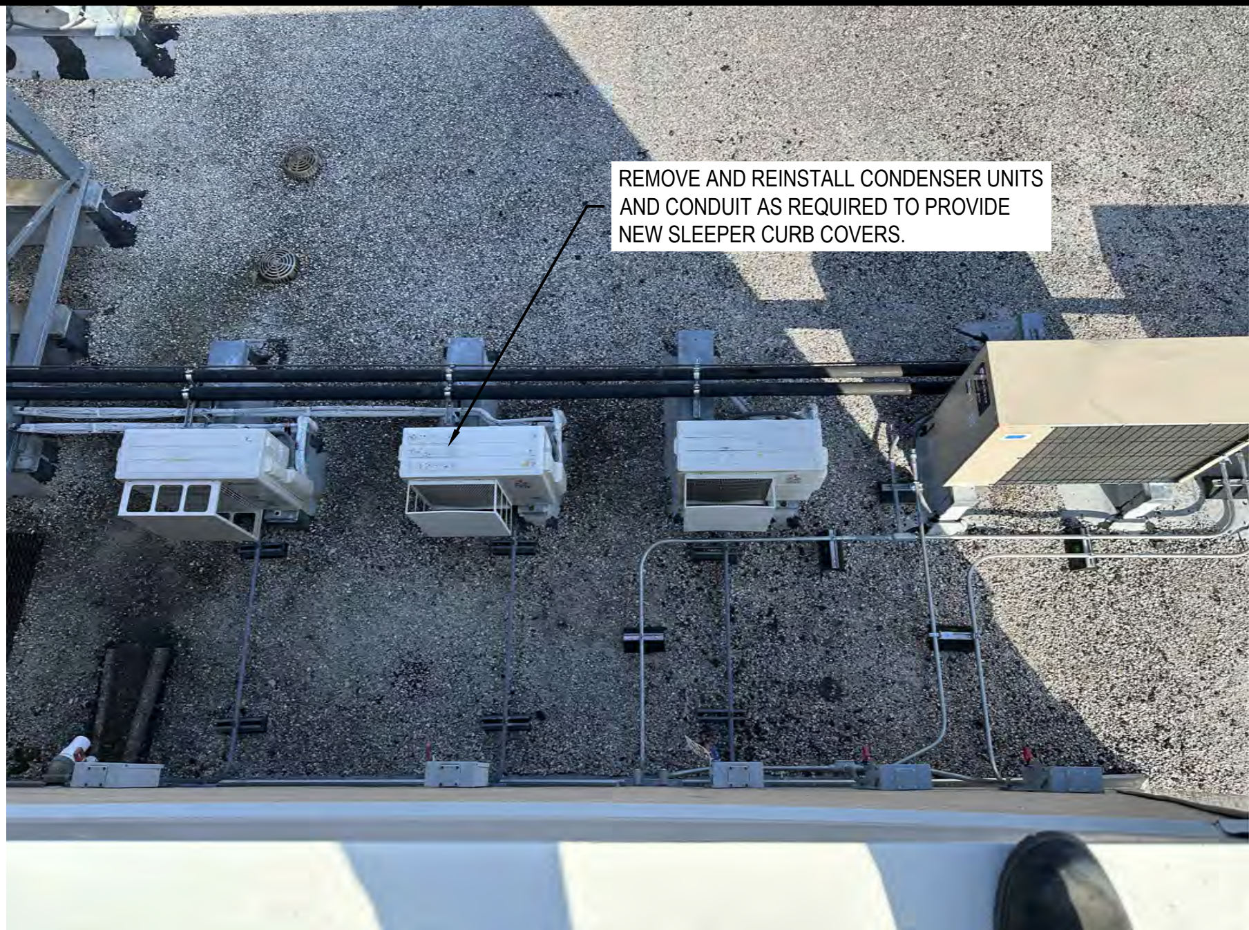
3 CONDENSER UNITS PH-01 SCALE: NONE
