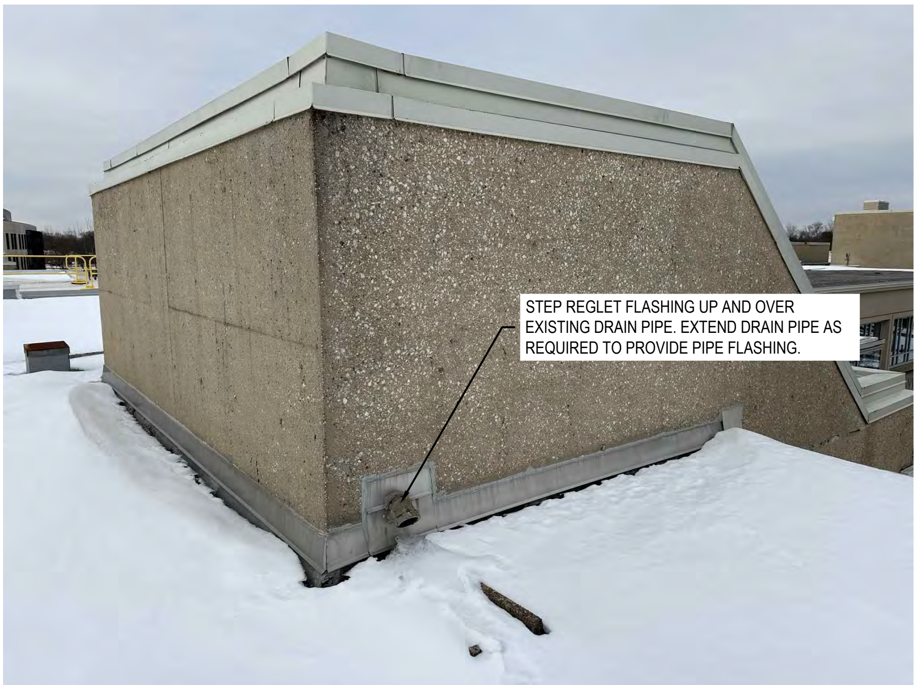
7 DRAIN PIPE PH-01 SCALE: NONE
