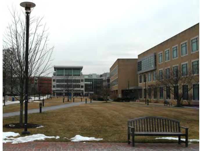
Main Quad view from Library to RCF
