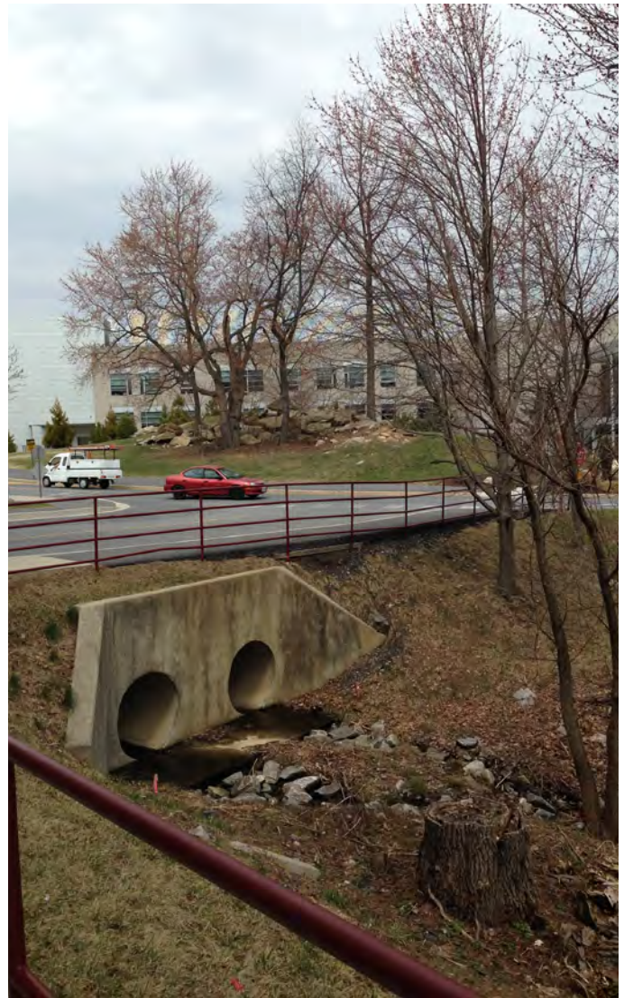
Storm Drain at Campus Drive
