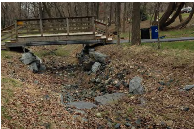
Pedestrian Bridge Over Stream
