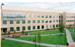
January 2003 Instructional Laboratory Building opens.
